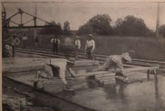
Finishing with Wood Floats.
